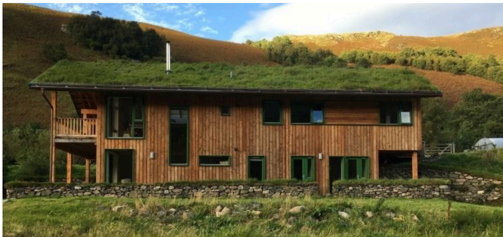
Figure 19- MAKAR construction in Glenelg
