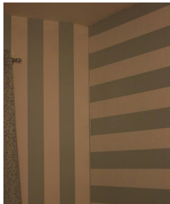
Figure 17: Bedroom 2 external wall/ceiling
