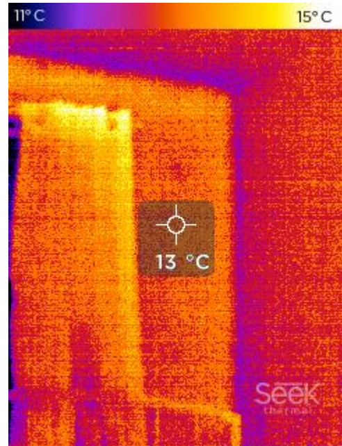
Figure 15: Bedroom 1 external wall/ceiling
