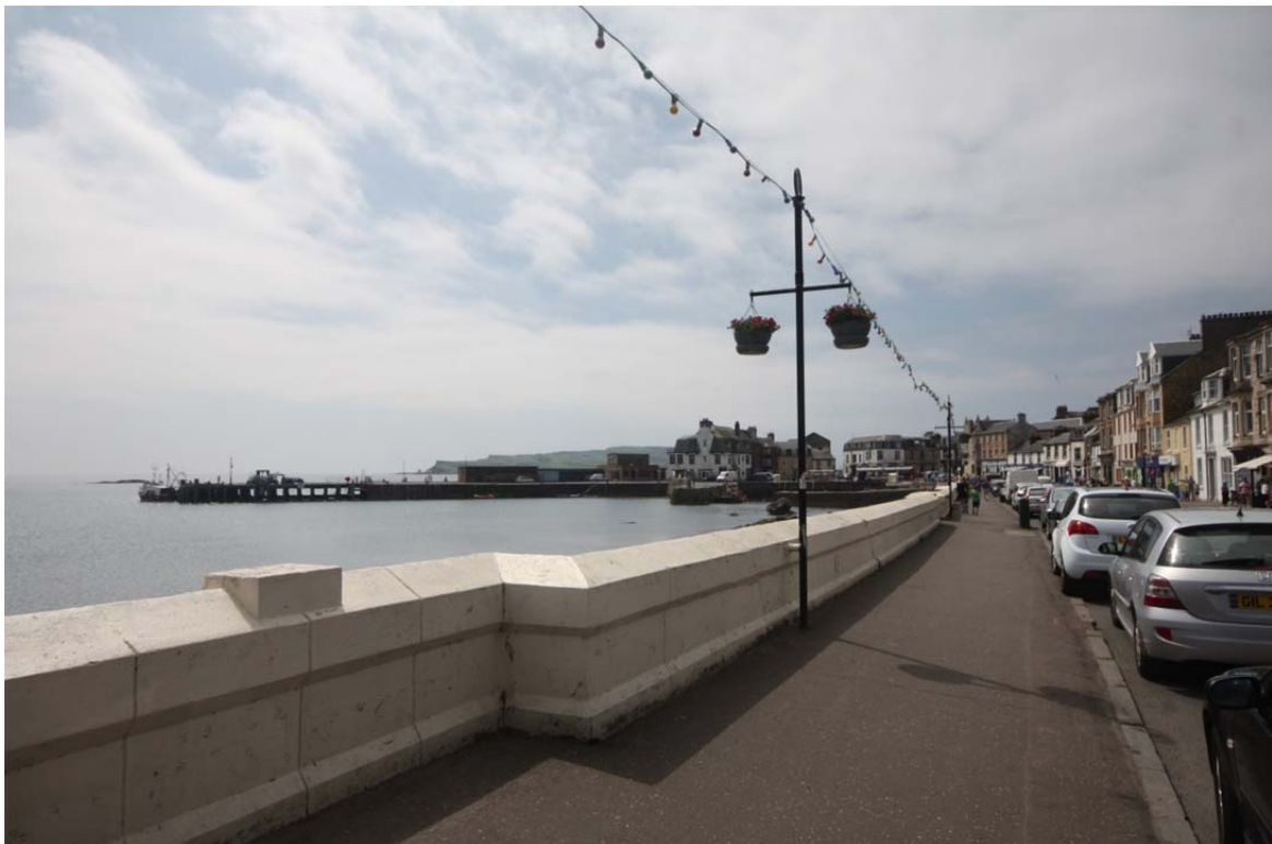
Figure 4-6: Stuart Street and Sea Wall July 2013, PDA
