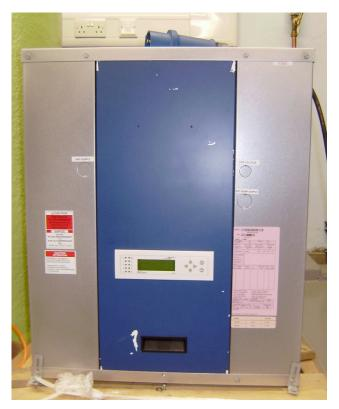
Figure 10: Waterfurnace EKW08 Ground Source heat pump.
