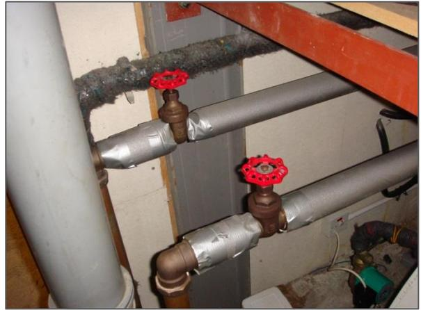
Figure 32: Partly insulated pipes
