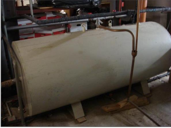
Figure 31: Uninsulated hot water tank
