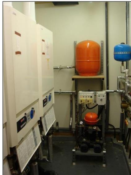
Figure 30: Gas boilers with expansion tank
