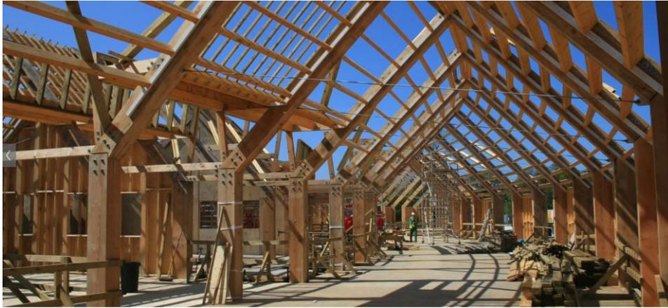
*Figure 6 The buildings timber frame during construction. (Page\Park, no date)*
