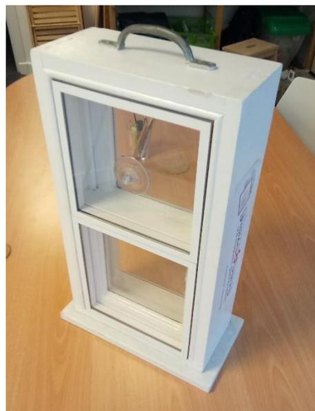
*Figure 68 - demonstrator of PVC secondary glazing installed by South Seeds*
