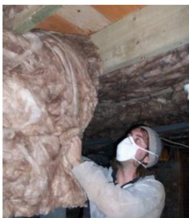
Figure 25 - South Seeds underfloor insulation
