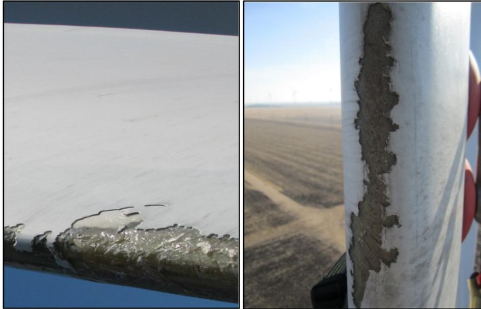
**Figures 13, 14:** Wind turbine blades and the erosion being present (Rempel, 2012),
