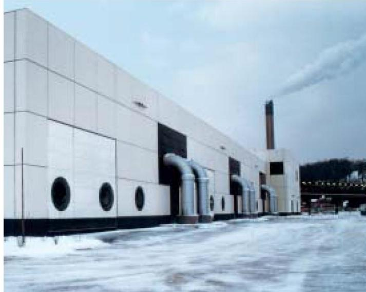
*Figure 16: Largest water heat pump in the world, Värtan Ropsten (Nowacki, 2014)*
