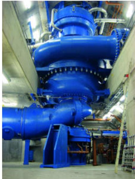
Figure 1 – Pump turbine in its turbine hall [5]
