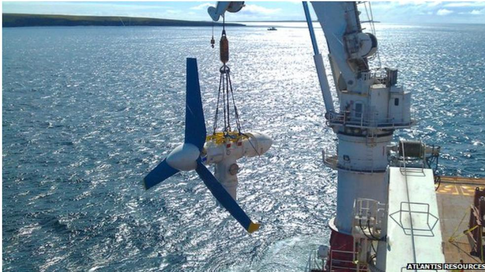
Figure 11 – Tidal stream turbines to be installed into the Pentland Firth [15]
