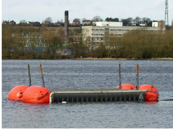
**Figure 2.9:** Flat plate heat exchangers at King’s Mill before being submerged (AWEB Supply, 2013)
