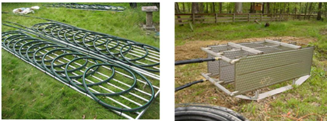
**Figure 2.5:** Heat exchangers for closed-loop surface water heat pumps. Coiled HDPE piping affixed to a steel frame (left) and Slim Jim™ flat plate heat exchanger (right). Images taken from (Wheildon's, 2012), (AWEB Supply, 2013).
