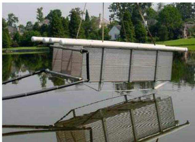
**Figure 2.6:** Four SJ-10T plates with inlet and outlet tubes (AWEBSupply, 2013)
