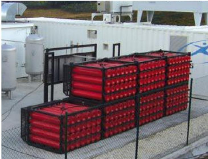
Figure 17. Pressurized hydrogen tanks installed in the experimental Wind-H<sub>2</sub> farm "Sotavento" (Rey, 2008)
