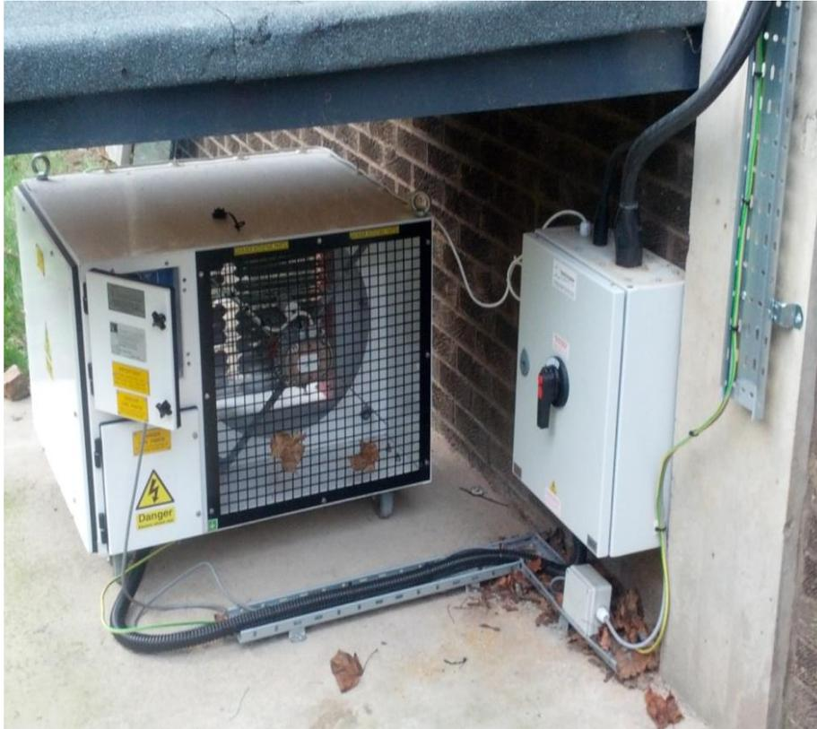
**Figure 9. 10.75 kW load bank**
