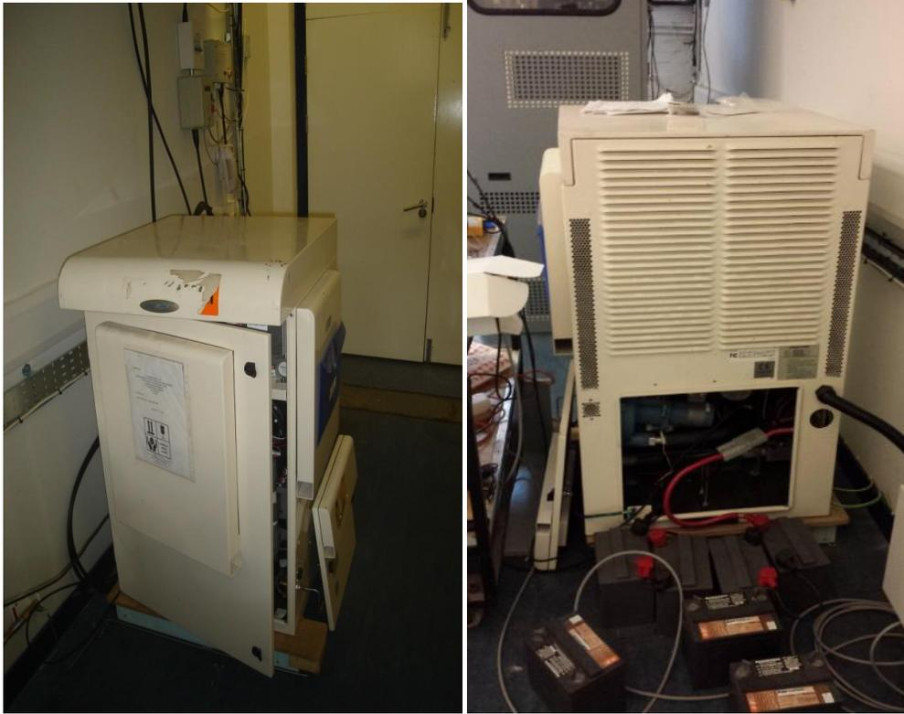
**Figure 6. GenCore 5B48 fuel cell**
