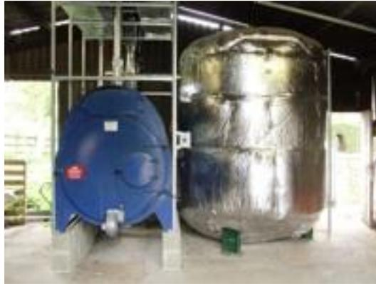
Figure 49: HT boiler composition (Teisen Products Ltd, n.d.)
