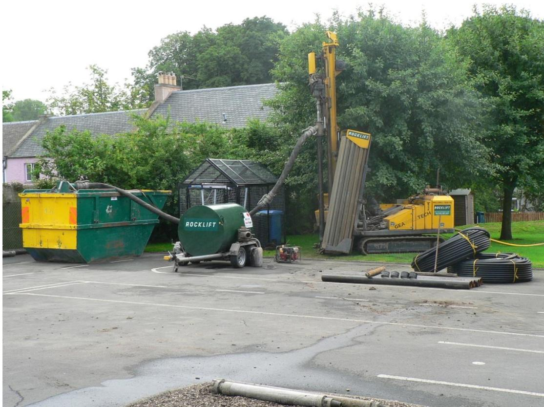
Fig 3.4.2 Clean drilling system (supplied by Rocklift Ltd)
