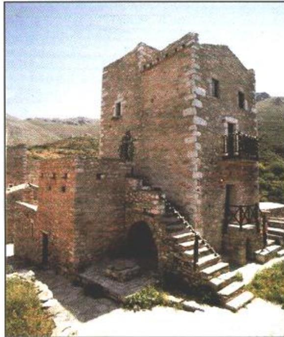
**Figure 2.3-3: Traditional building in Mani, Greece, with heavy structural elements and very good thermal behaviour during the summer period [9]**
