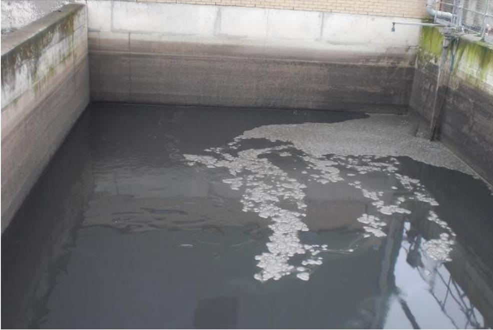
**Figure 14: Digested Sludge Storage Tank**
