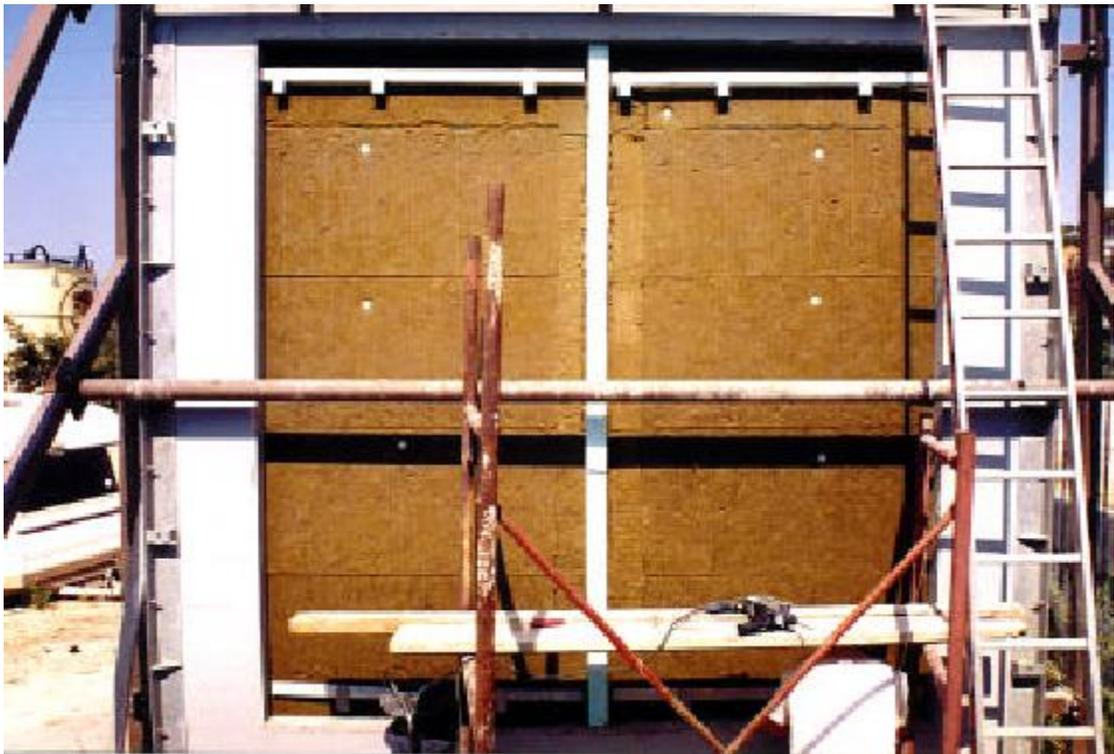
*Figure 18<sup>[VI]</sup> – Positioning of the insulation layer between the two parts of the wall components*
