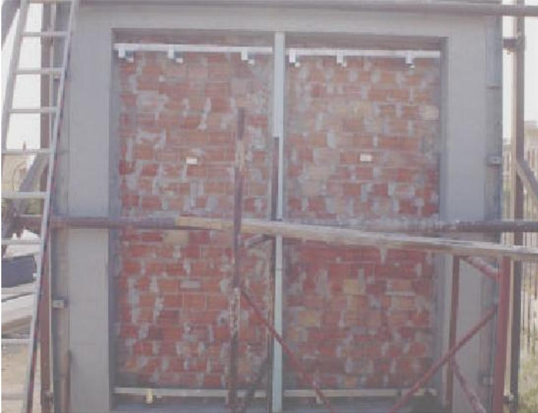
**Figure 17<sup>[VI]</sup> - Positioning of the special metal support elements for the fixing of the prefabricated concrete slab**
