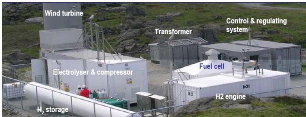
**Figure 14: Equipments of Utsira demonstration project [21]**
