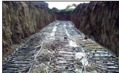
Fig 23b. Slinky Pipes in a Trench [16]
