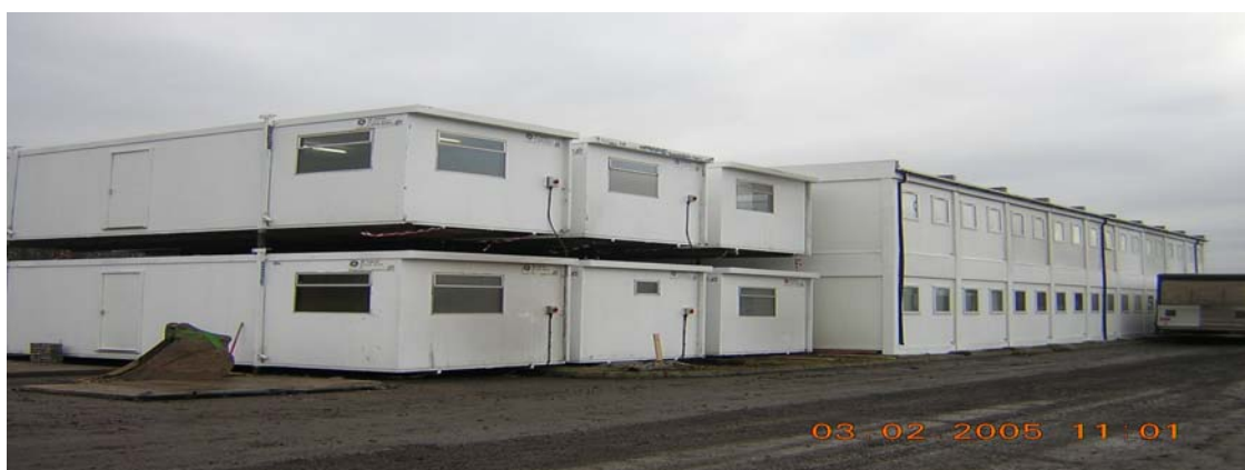
Figure5: NATS cabin accommodations
