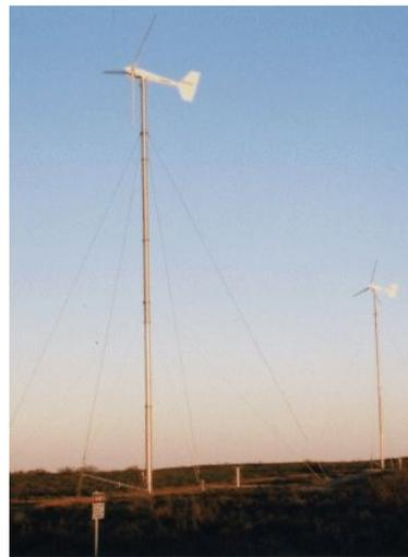
Figure 5.4: 20 kW Westwind turbines at Exmouth, Australia
