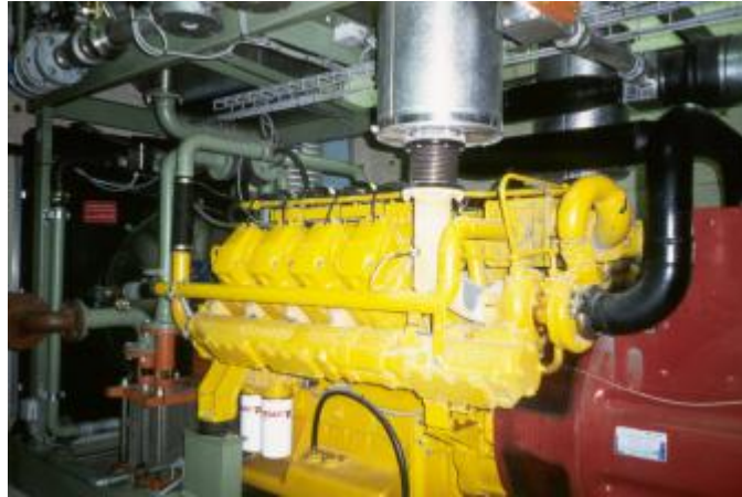
figure 9. Biogas use in internal combustion engine
