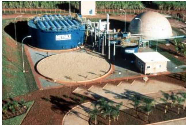
figure 5. A digester treating dilute wastewater at a fuel ethanol production plant in Brazil
