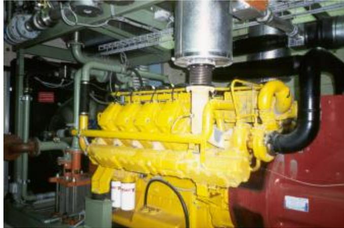
**figure 9.**Biogas use in internal combustion engine
