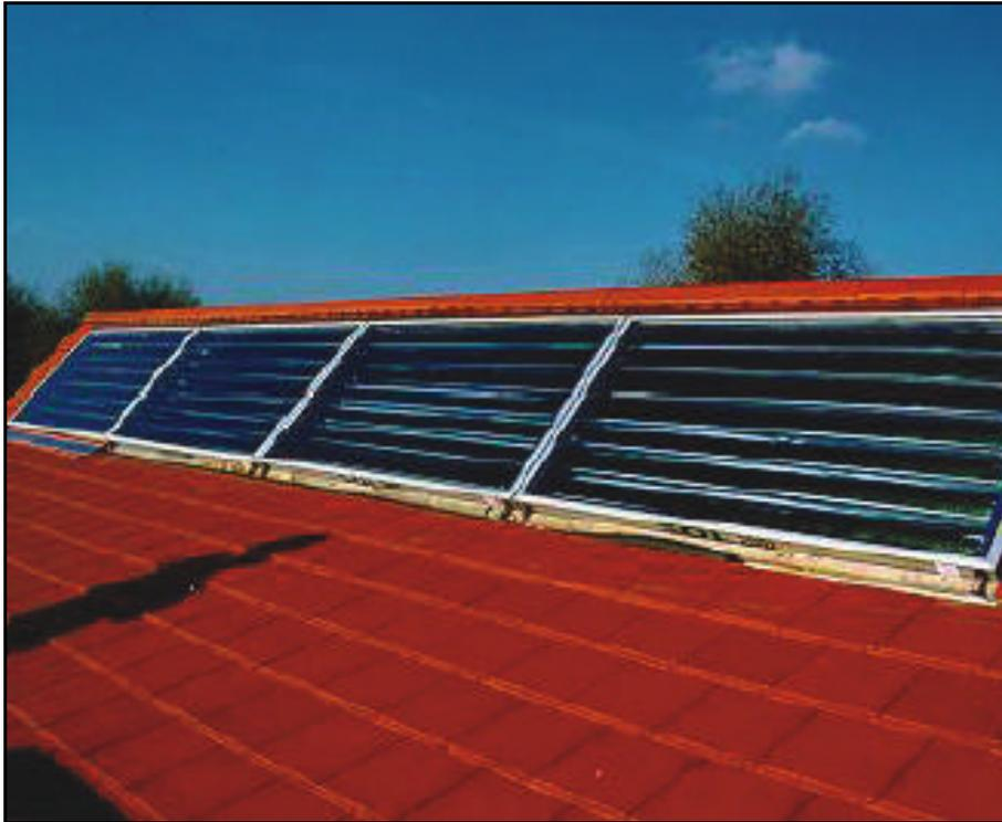
Figure II-11 example of compound parabolic collectors in Portugal [13]
