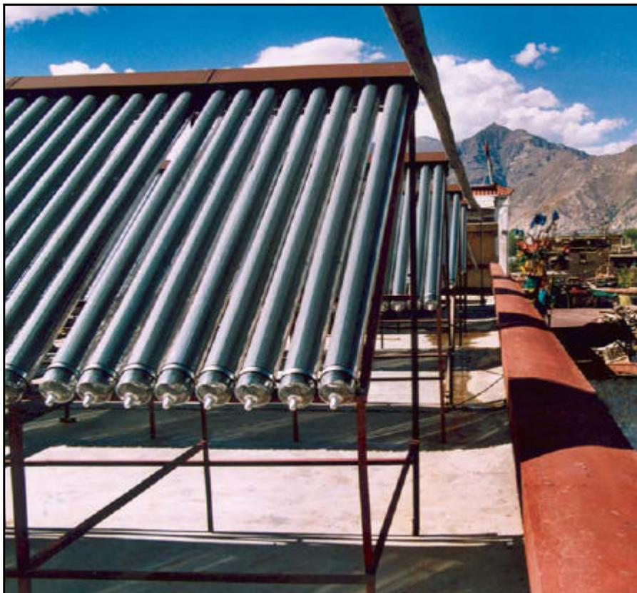
Figure II-12 example of evacuated tube collectors in Tibet [14]
