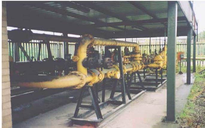
Figure 18 - Photograph of a mains gas pressure reducing station.
