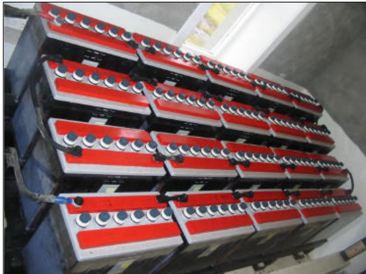
**Figure 9 - Battery bank installed on Muck**
