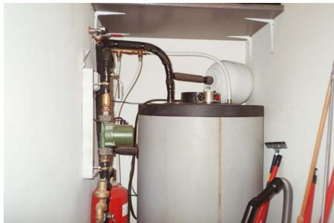
Figure 5.6.8.2.2: Domestic hot water system with a deposit of 3 litres located in small room inside the house
