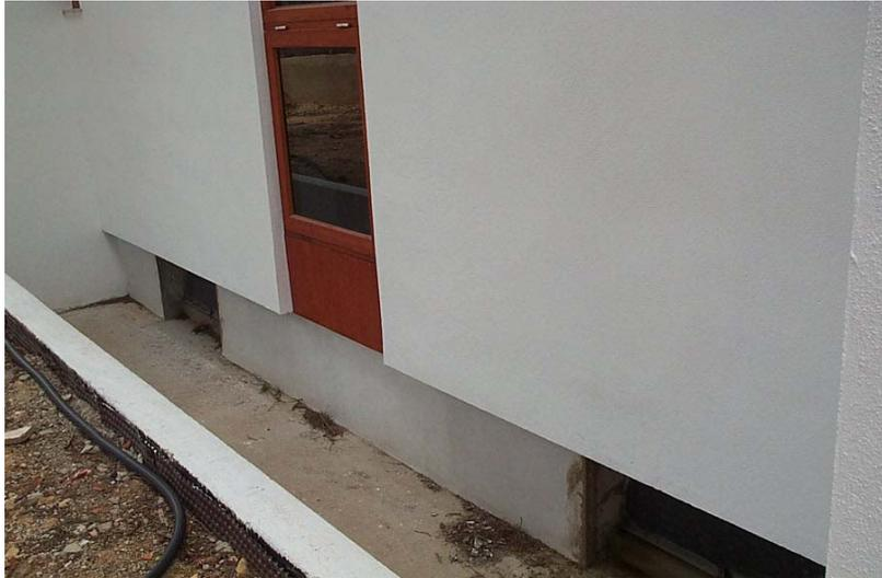
Figure 5.6.6.3: Detail of the ventilation system. Project of Luis de Garrido architect
