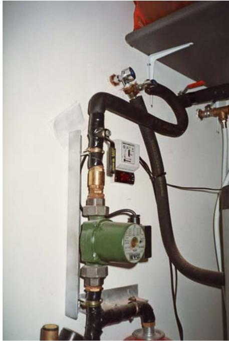
Figure 5.6.8.2.1: Temperature control system. The small screen shows 84 °C.
