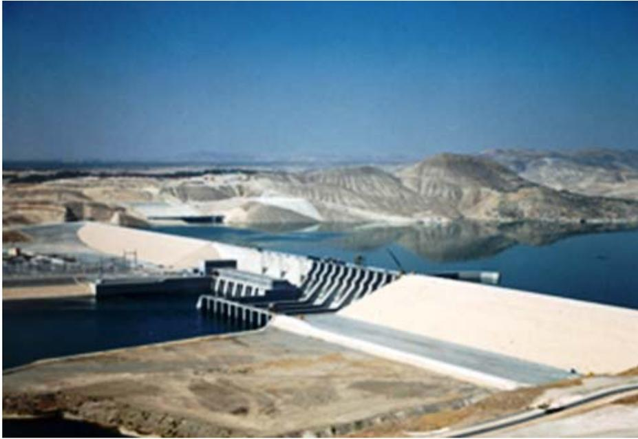
Figure 43. Concrete Gravity Type - Birecik Dam on Euphrates River, Turkey.
