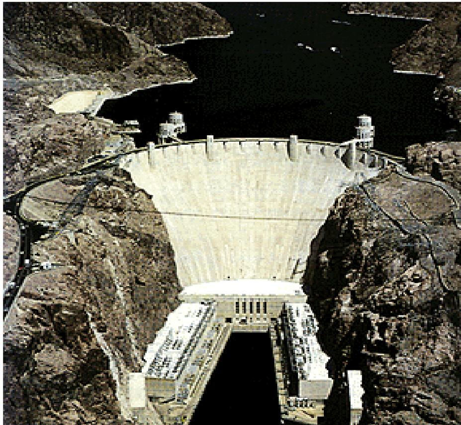
Figure 44. Concrete Arch Type - Hoover Dam on Colorado River, U.S.A.
