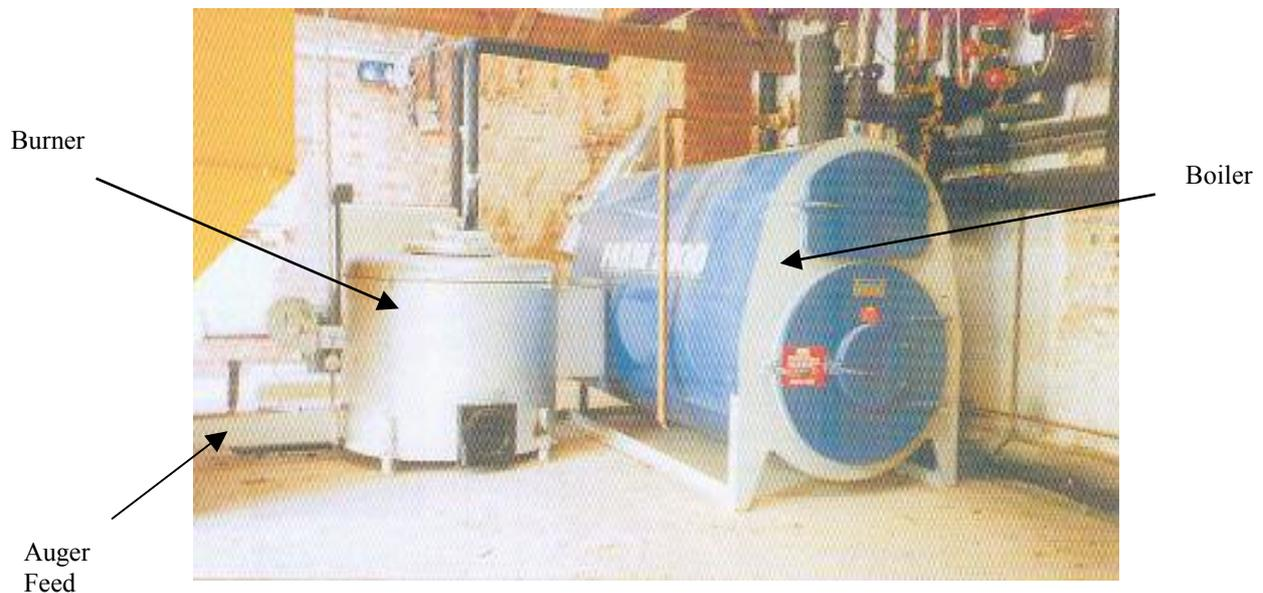
Fig. 32(a): A woodchip boiler system (pre-combustor design: see also 5.4.1.4) [23]
