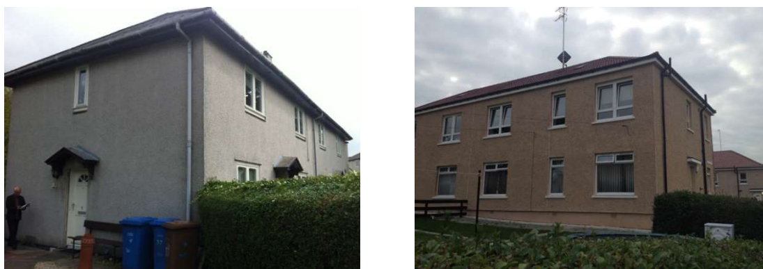
Figure 2: A typical uninsulated property in Carntyne (left) and an externally insulated property in Shettleston (right).
