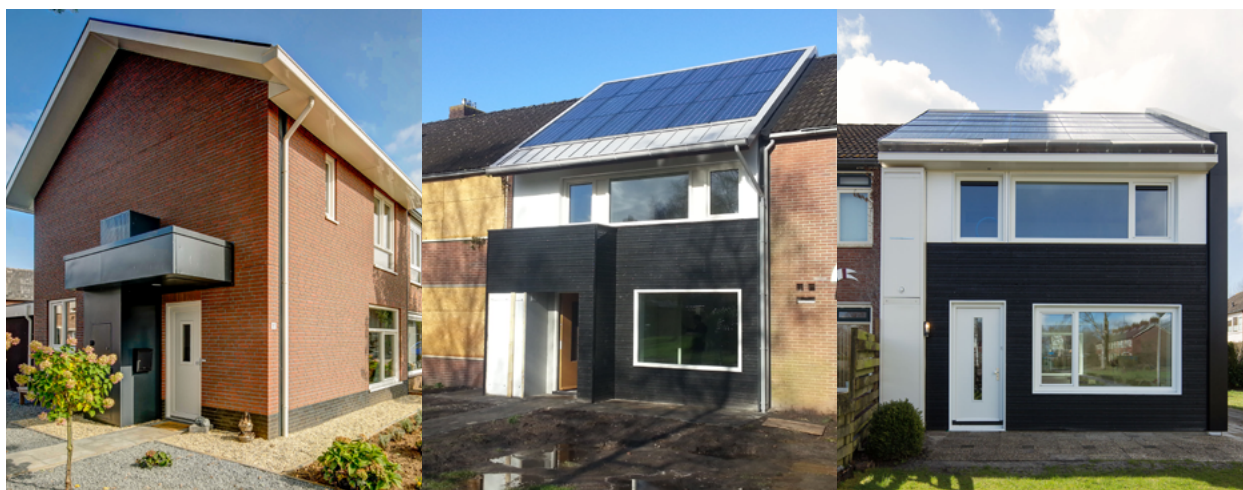
Three prototype versions from one company (Volker Wessels): Version 1, (Dec 2013, left) took 2 weeks to place and has the energy module sticking out; version 2 (middle) took 1 week and has the energy module more integrated around the front door. Version 3, (February 2015, right) took 1 day and has the module integrated in the façade. Cost reduction between version 1 and version 3 is ±30%. Watch the movie of the 1 day refurbishment here: https://www.youtube.com/watch?v=I3WBT2eAArI
