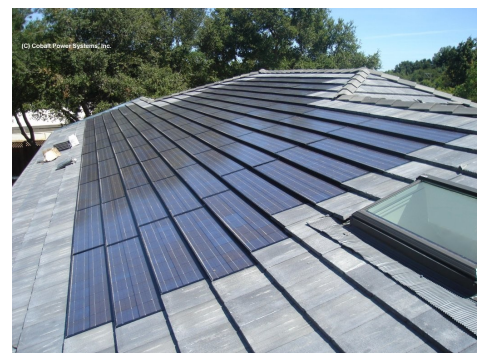
Fig: Integration module roof tiles
