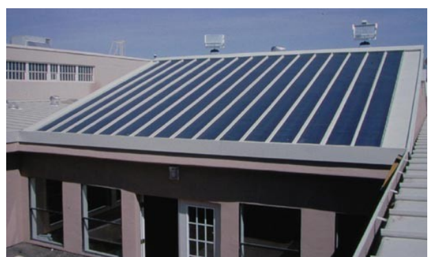
Fig: Integration module roof tiles
