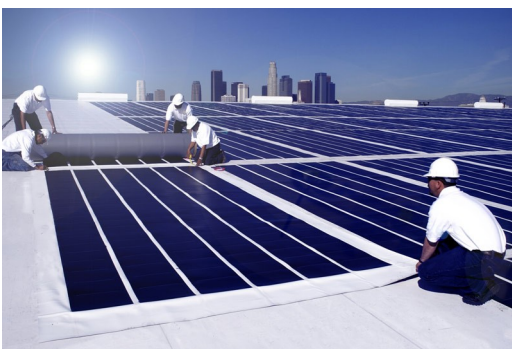
Fig: Thin film solar cell integration for flat roofs
