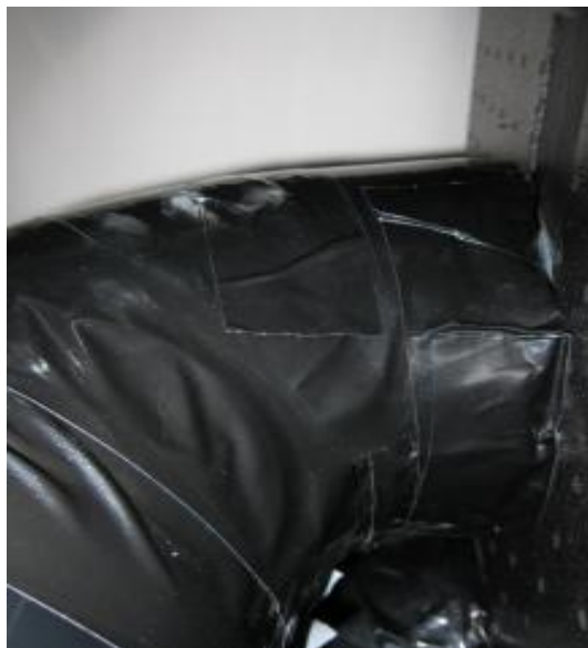
Figure 6.26 – Remedial work to MVHR ducting. Further improvements required so that PassiveHouse standards are met
