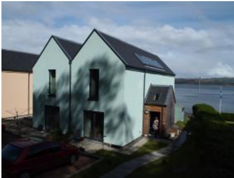
Figure 6.17 - Dunoon PassiveHouse – Note Solar Thermal Panel Installation
