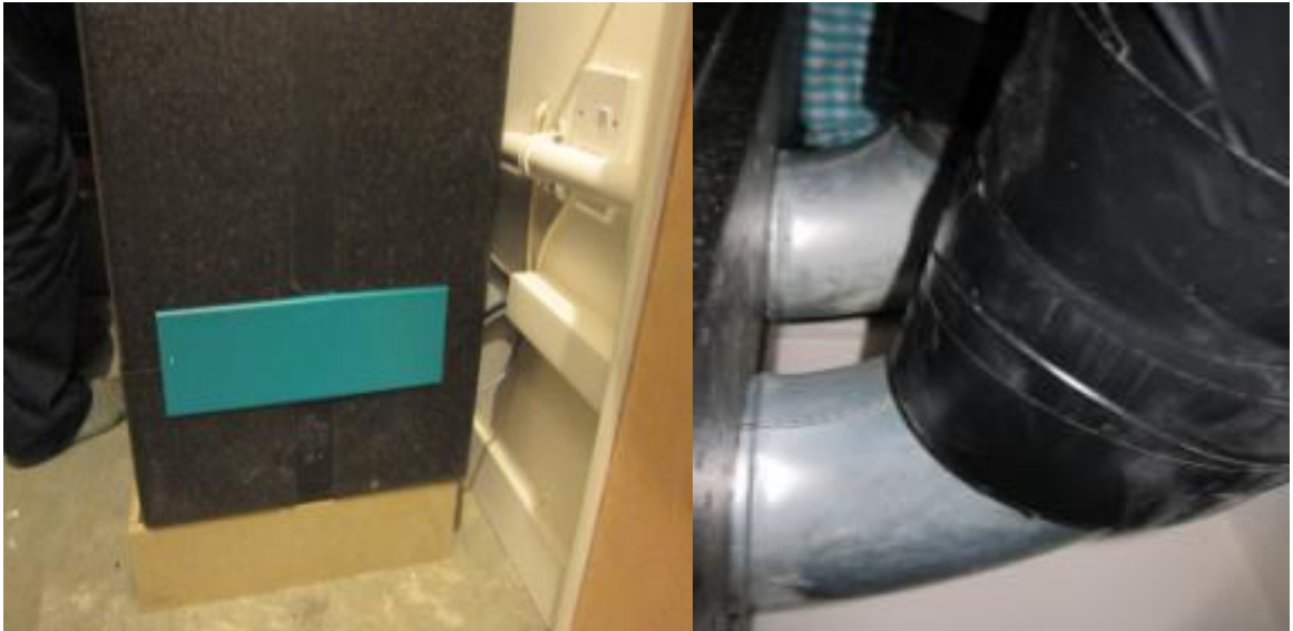
Figure 6.22 – PassiveHouse MVHR Ducting Unit; insulation issue
