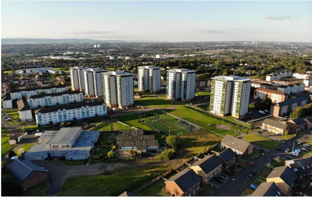
Figure 6.1: Panoramic view of WWHC with the 6 high rise towers and 5 low rise blocks
