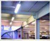
This LED light fitting has been manufactured from corrosion resistant glass reinforced polyester and contains a
