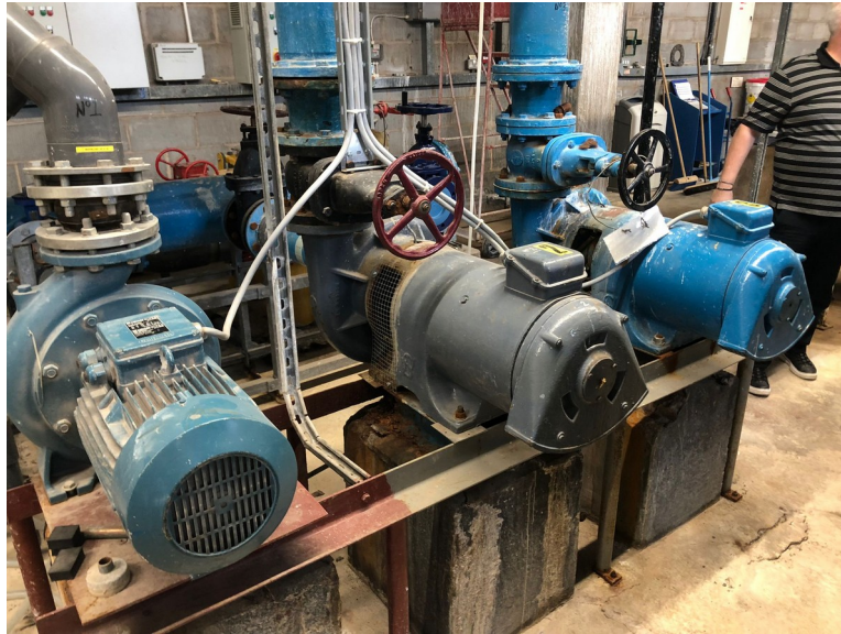
Figure 1: Main pool water pumps (Photograph taken on site visit in July 2024)
