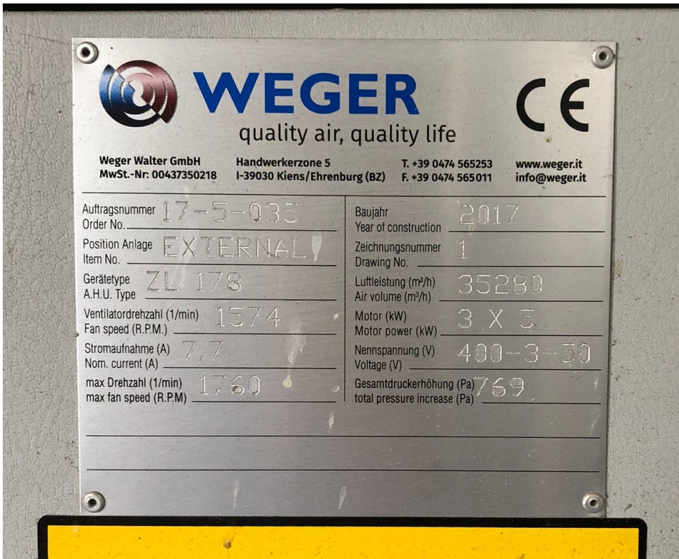
Figure 28: Citadel AHU nameplate
