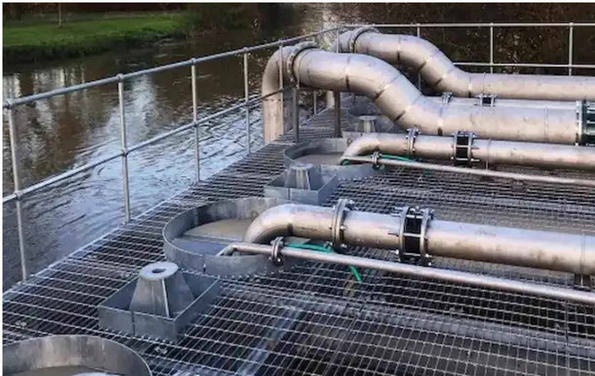
Figure 12: Abstraction equipment for an open loop water source heat pump (ACR Journal)
