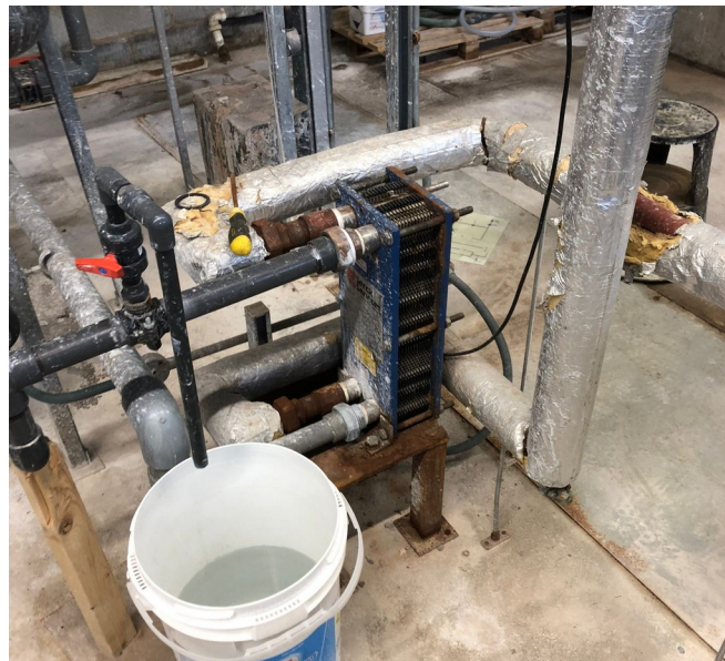
Figure 2: Plate heat exchanger for the diving pool (Photograph taken on site visit in July 2024)
