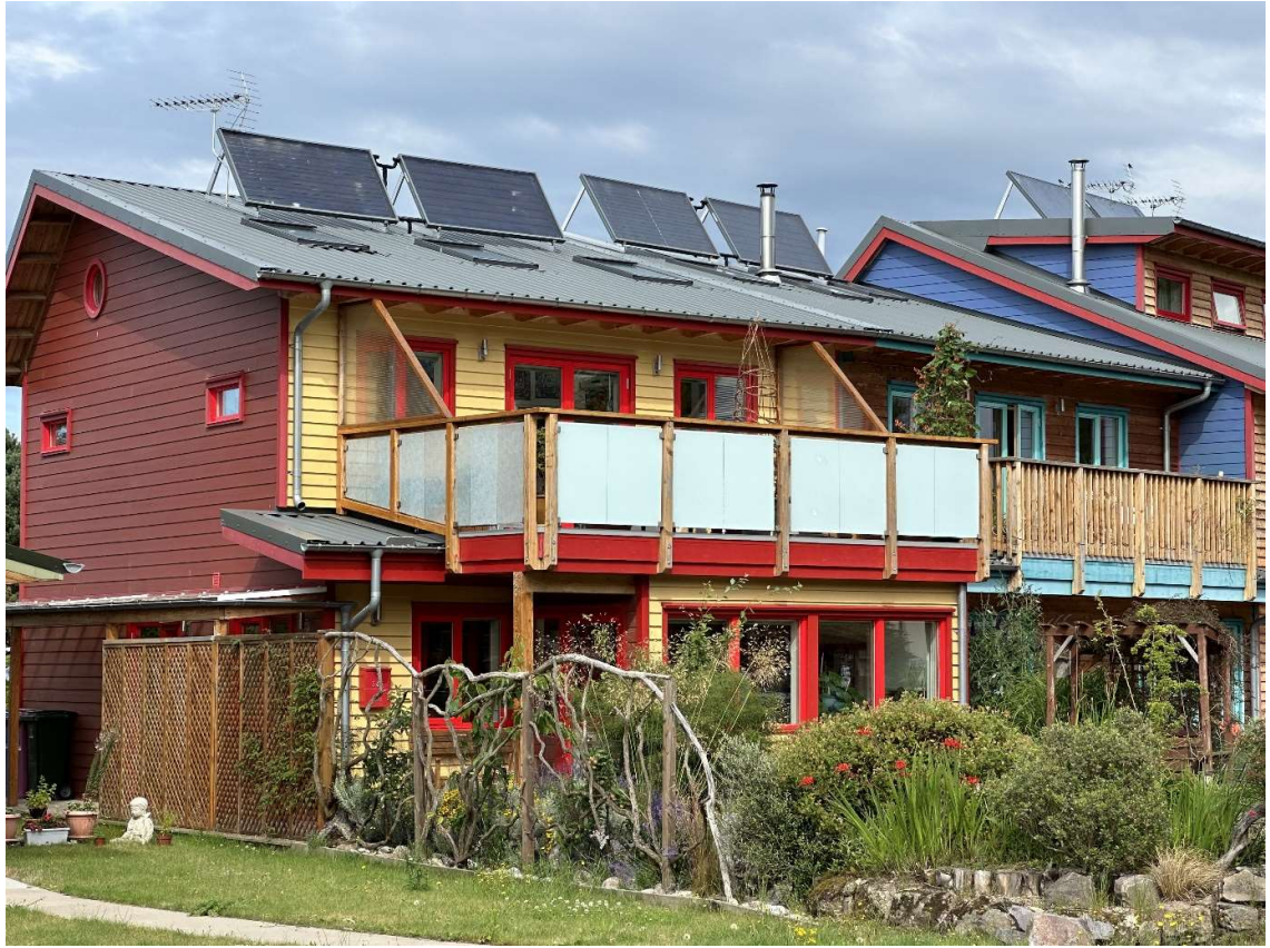
Figure 2: Findhorn Social Housing with Heat Pump, PV and Solar Thermal
