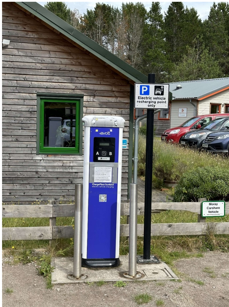
Figure 3: 22kW Fast Charge EV at Findhorn
