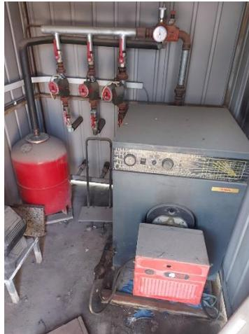
Figure 29: Oil condensing boiler and equipment.
