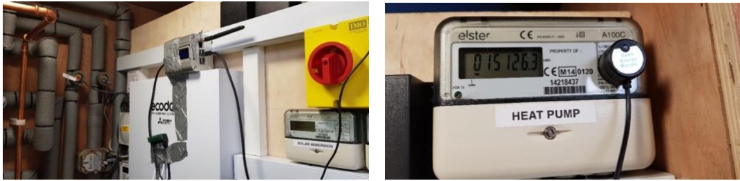
Figure 10: emonPI hardware and energy meter pulse input to heat pump at WW (3)
