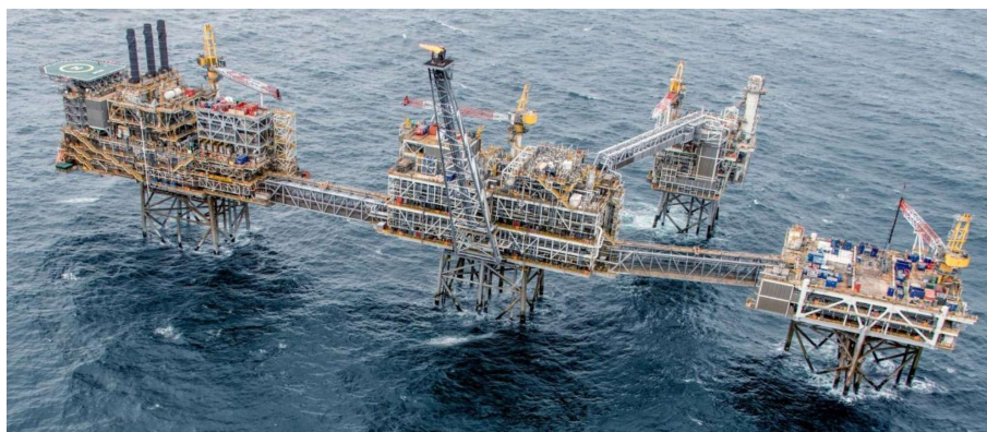
Figure 6: Buzzard Field surface infrastructure of four BLPs [57].
