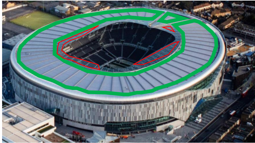
Figure 29: Aerial view of The Tottenham Hotspur Stadium, with areas of the stadium roof suitable to hold PV panels shown in green and unsuitable areas shown in red.
