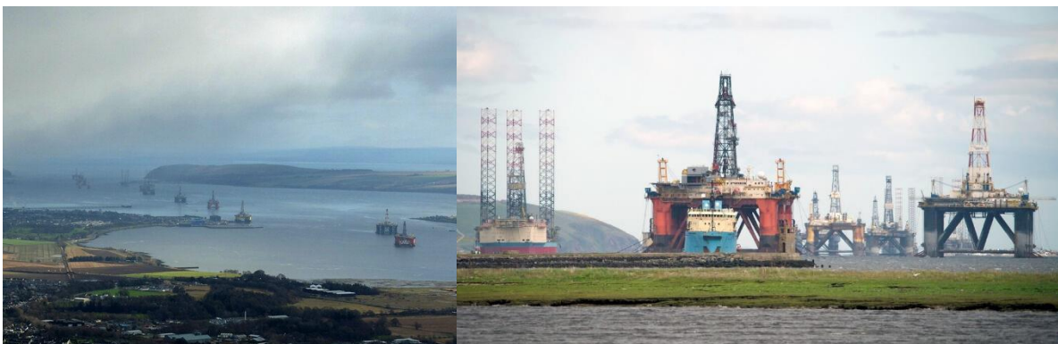
Figure 9: Abandoned oil rigs in the Cromarty Firth, in the north of Scotland. [79]
