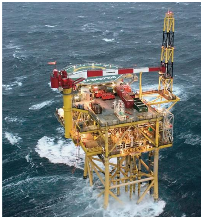
Figure 12: Shell's Goldeneye platform [112].
