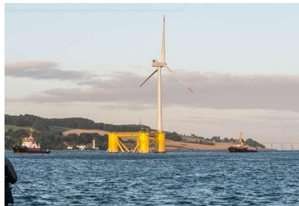
Figure 3: A floating offshore wind turbine in the Kincardine Offshore Windfarm 15km off the Aberdeenshire coastline. An example of the type to be used in the Dolphyn project. [16]
