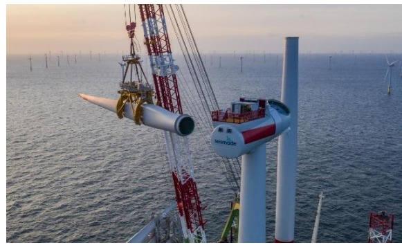
Figure 6: Installation of blades at SeaMade, Belgium's largest offshore wind farm [52]
