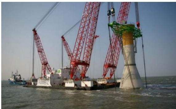
Figure 7: Installation of GBS support structures in Thornton Bank offshore wind farm [51]
