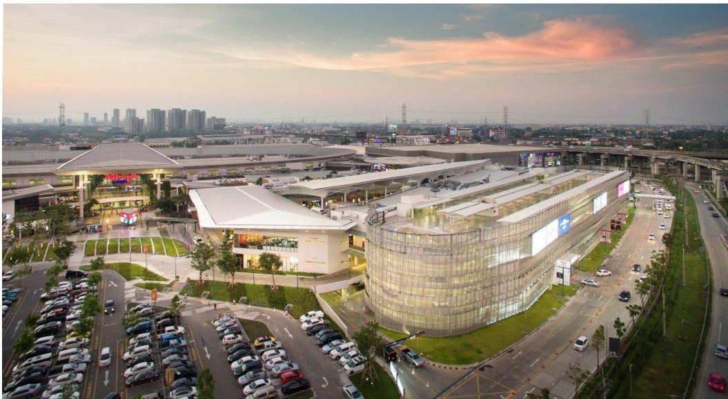
Figure 5.1 : View of the Megabangna Shopping Centre (Source: Matichon News)
