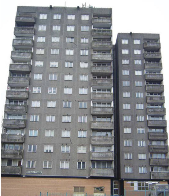
Figure 2: Higher-rise tower block at WWHC before efficiency upgrades (d+b facades, 2011)
