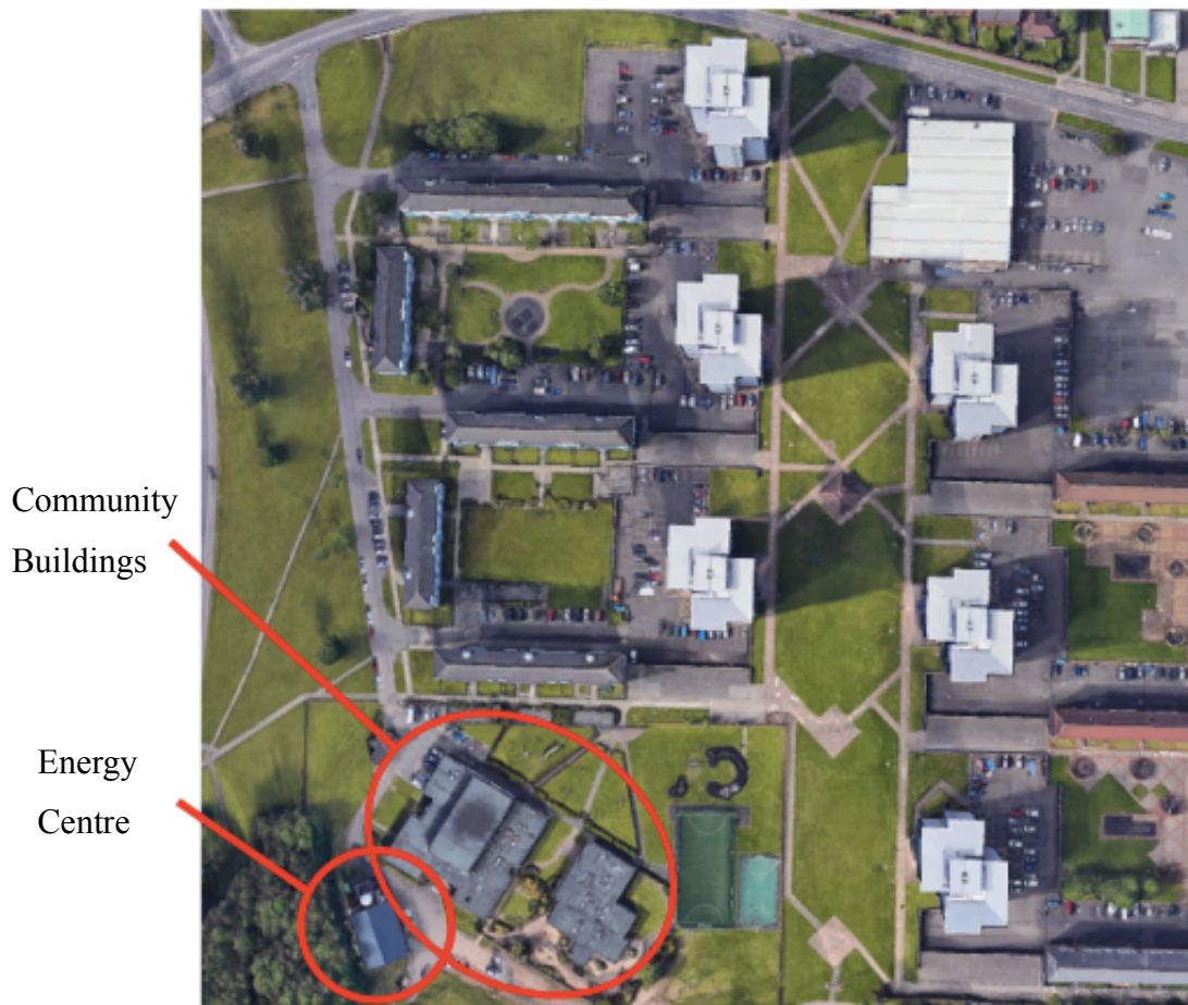
Figure 11: Aerial view of WWHC, community buildings and the energy centre are highlighted beside the residential buildings
