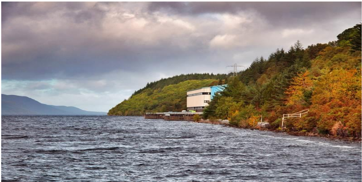
Figure 6 - Foyer's Pumped Hydro Station
