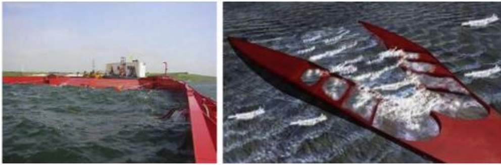
Figure VII: WaveDragon Overtopping Converter (left) and the WaveCat Overtopping Converter (right). (Pérez-Collazo, Greaves and Iglesias, 2014).
