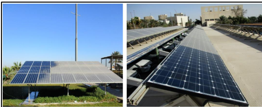
Figure 3-2: before and after cleaning PV modules at different locations in Kuwait.
