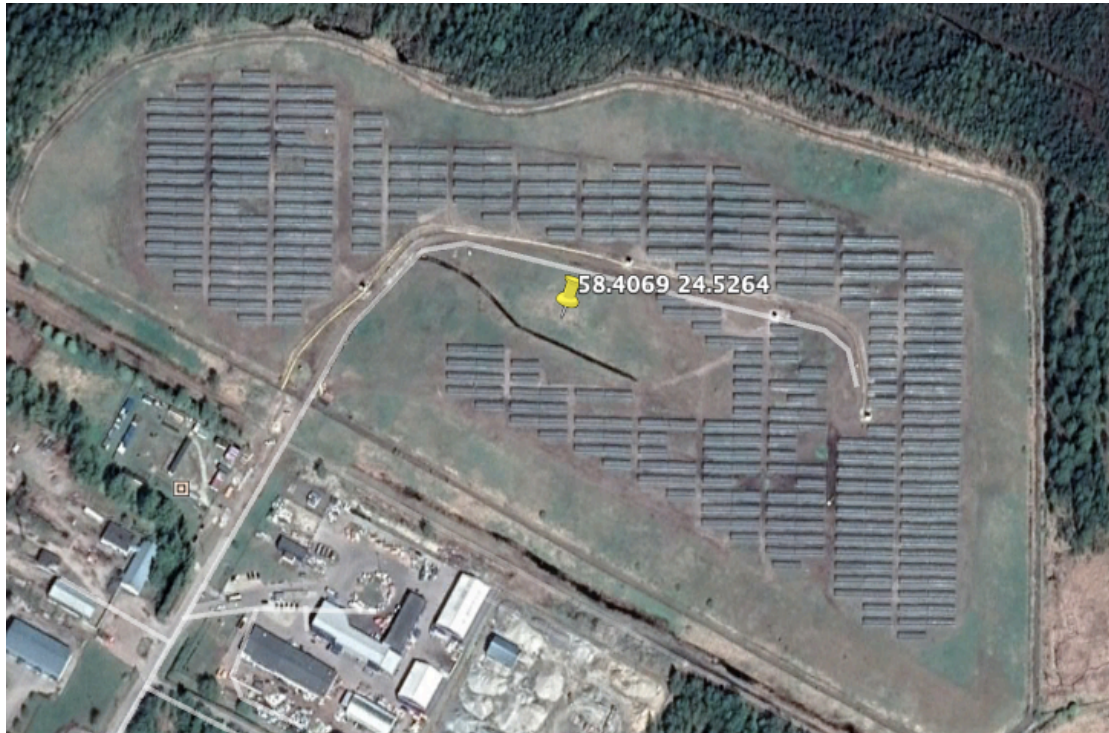
Figure 24. Aerial photo showing the layout of the Pärnu Päikesepargid PV plants.
