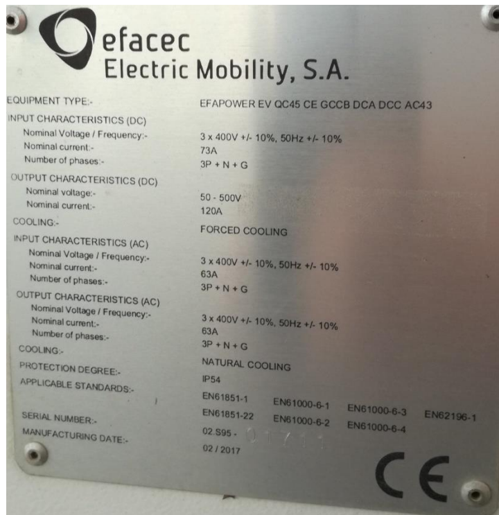
Figure 3: Technical Specifications of the EFACEC fast charger.
